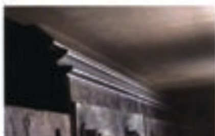
4. Spring time. A high-performance bellows seal in flex position, contacting the sector plate. Courtesy: Paragon Air Heater Technologies
